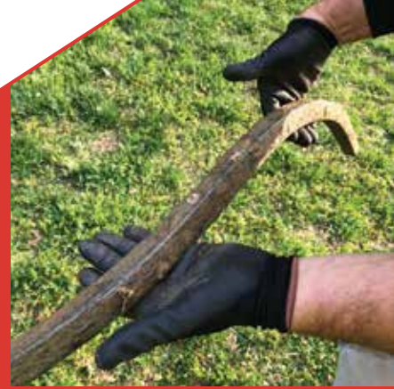
Most of the underground obstructions that crews encountered were due to as-builts that did not document footers for barracks.
