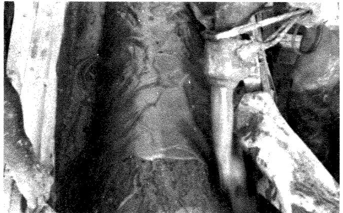
Ultra-Lite insulates steam duct to conserve energy. — Scarborough, Ontario
