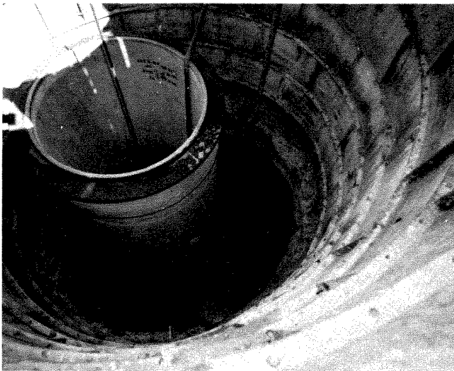
Ultra-Lite 400 was used as a shock absorbing annular fill to protect a water transmission line from damage from future rock blasting. — Austin, Texas
