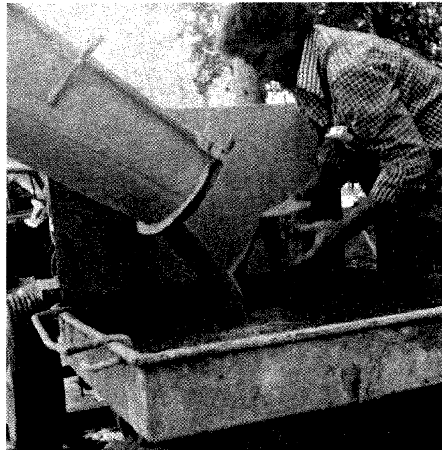
Licensed contractor checking density to verify conformance to specification.
